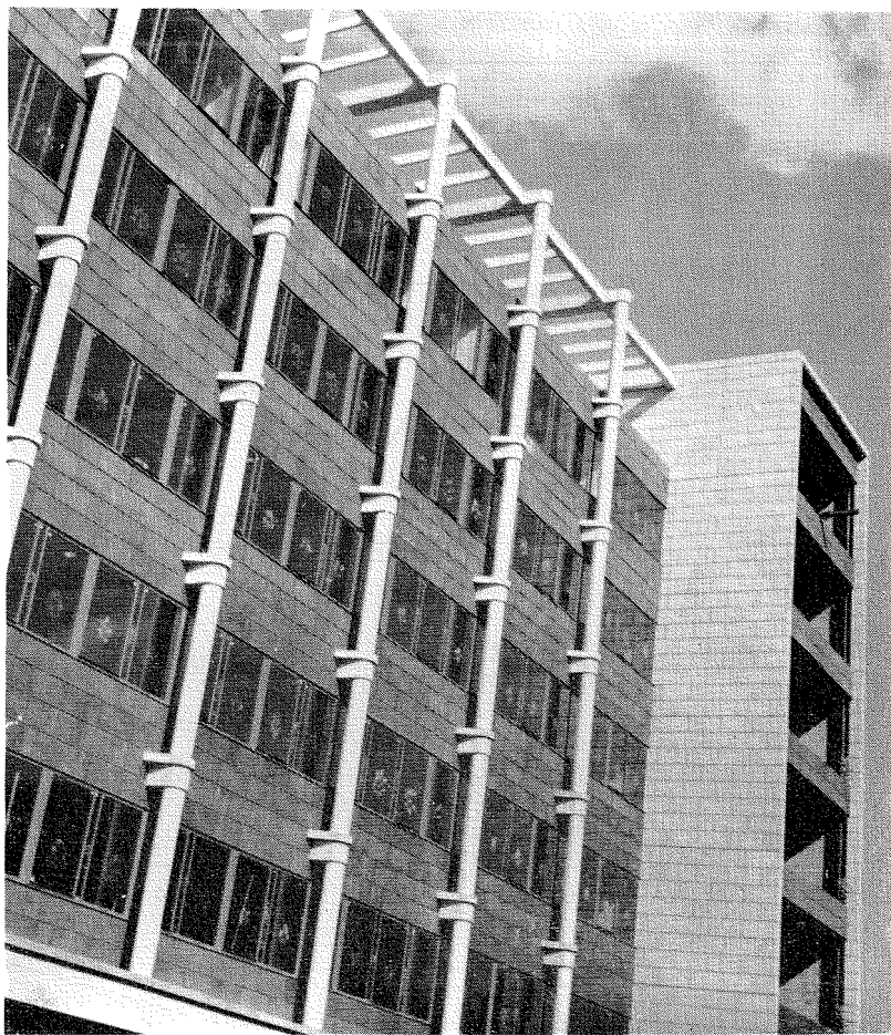
Fig. 17.—Military Hospital, Copenhagen. The Columns were Precast.
