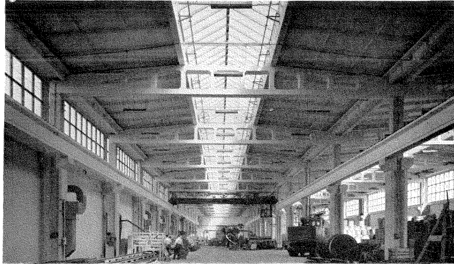
Fig. 19.—Factory with Precast Columns and Prestressed Beams.
